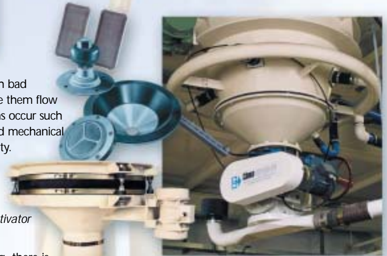
■ Silo discharge system with fluidisation and rotary valve
